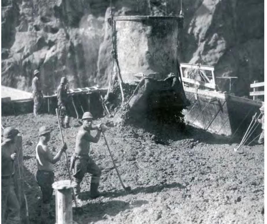
First bucket of concrete for Hoover Dam placed in June 1933
