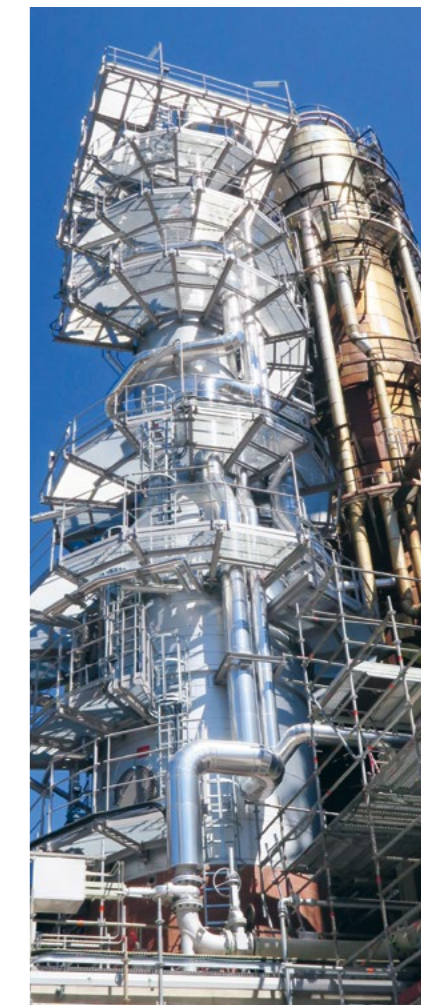
Neue Pre-Flash-Kolonne in Cressier.
